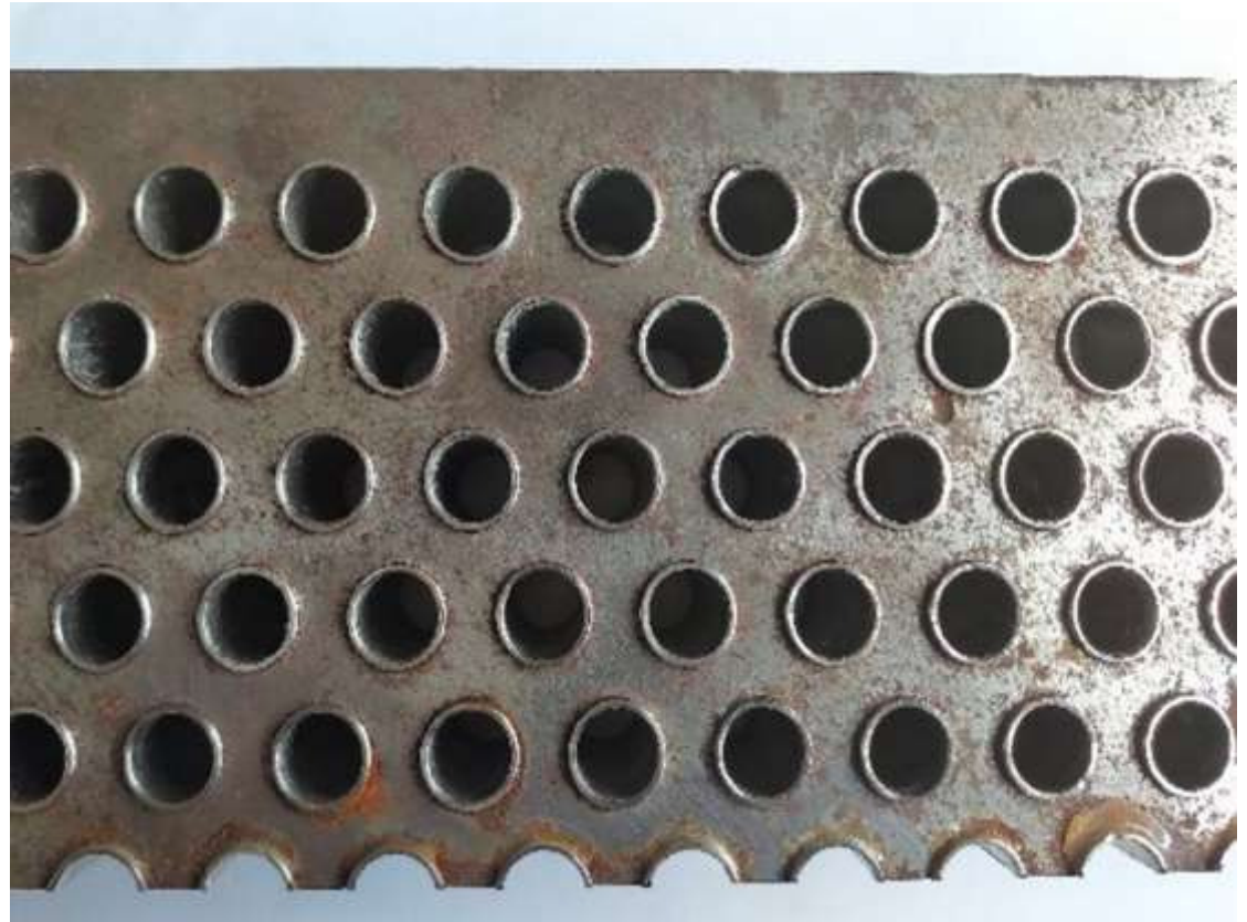
Unprotected Nuclear steel tube sheet manufactured in 2008
